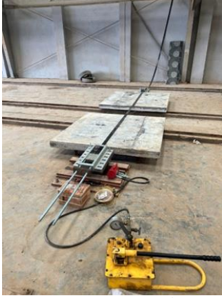
Fig. 2 Pre-stressed processes of CFRP tape
