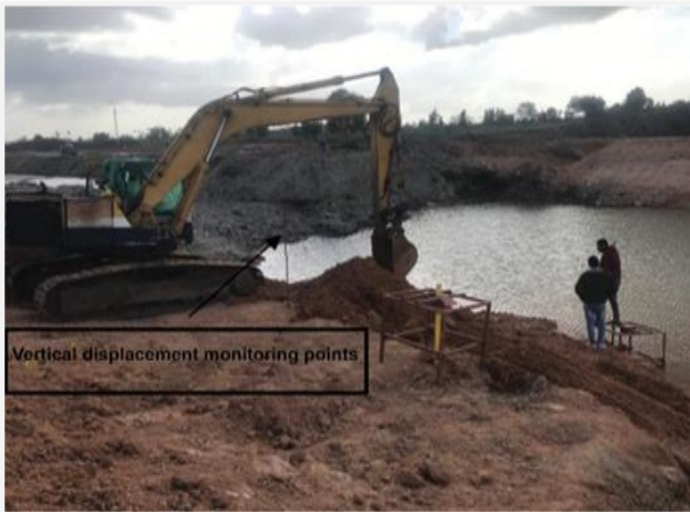
Fig. 5 Field locations of vertical displacement monitoring points at the site
