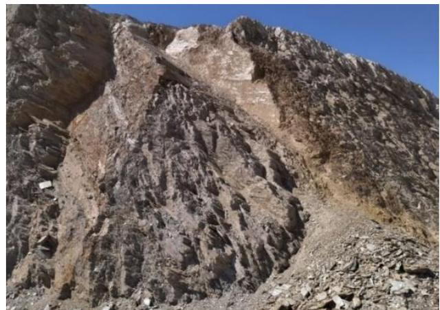
Fig. 12 Several detached blocks are observed in section 11
