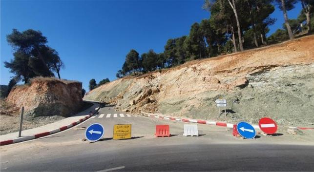
**Fig. 2** Instability of a rocky slope in northern Morocco; the road has been diverted due to these instabilities
