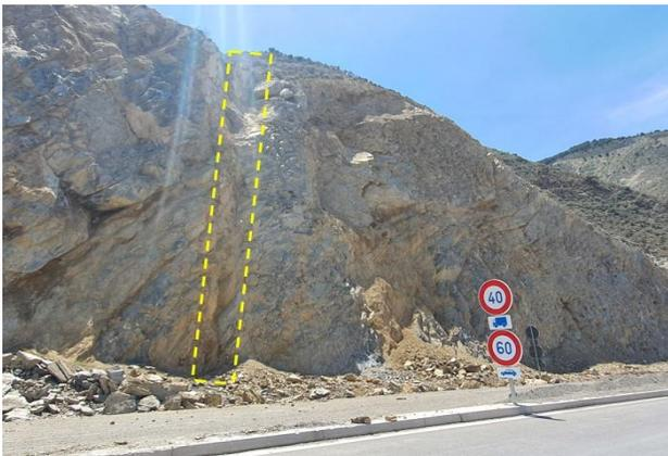
Fig. 11 Weak plane in the form of a marly joint
