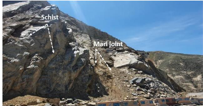
Fig. 6 Slopes dominated by schist and marly schist
