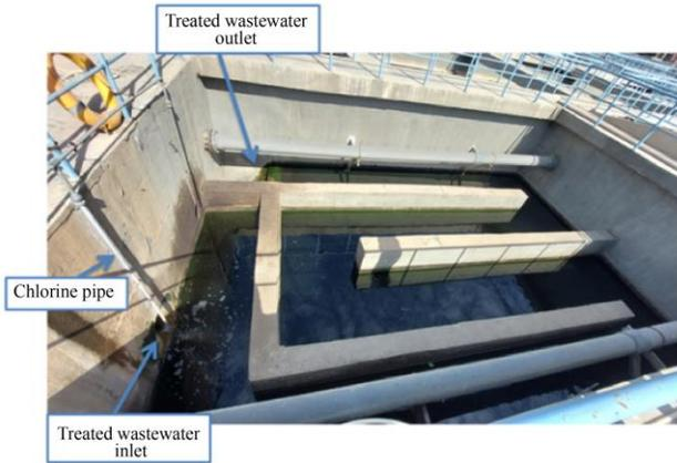
Fig. 10 Disinfection contact tank
