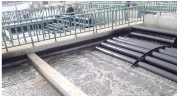
Fig. 2 Modified rotating biological contactor
