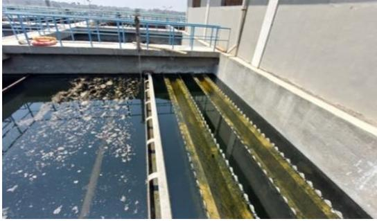
Fig. 5 Sedimentation tanks outlet channels
