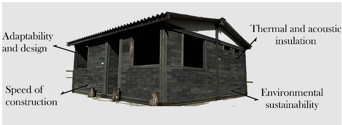
Fig. 7 Prototype house constructed from recycled plastic bricks
