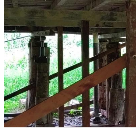
Fig. 5 Method of raising the height of the stilt house pillars using the dovetail joint technique
