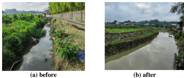
Fig. 10 Normalization of the Sempaja River carried out by the Government in 2021
