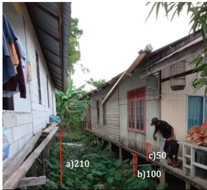
Fig. 3 Adaptation of stilt houses: a) less than 10 years and floor height 210 cm b) 10-20 years and floor height 100 cm c) Flood height more than 40 cm above the floor
