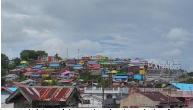
Fig. 1 Typical zinc roofs in Manado, Indonesia, predominantly appear in three color variants: blue, maroon, or unpainted silver, reflecting common local practices in roofing material finishes
