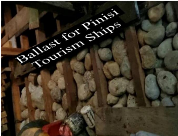
Fig. 3 Construction of pinisi
