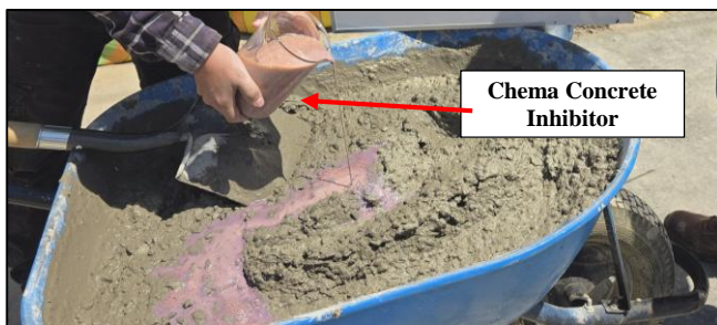
Fig. 10 Application of the corrosion inhibitor scheme in concrete
