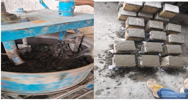
Fig. 8 Concrete mixing and mould preparation
