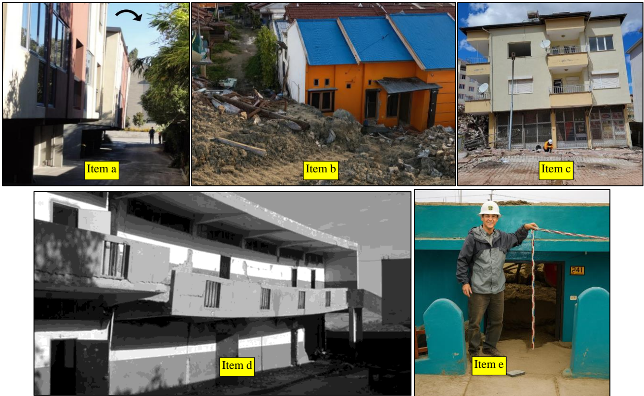
Fig. 1 Cases of soil liquefaction
