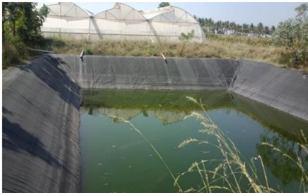
Fig. 2 Lined farm pond with polythene
