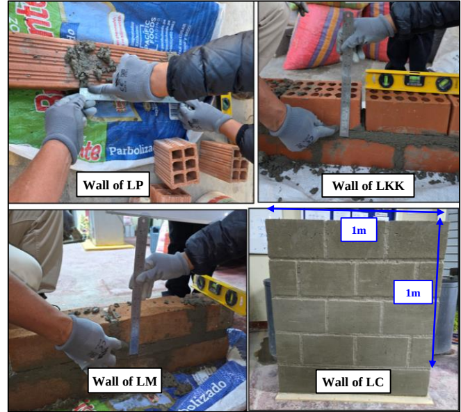
Fig. 12 Bricklaying
