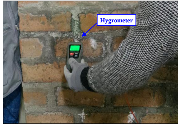
Fig. 15 Initial moisture measurement
