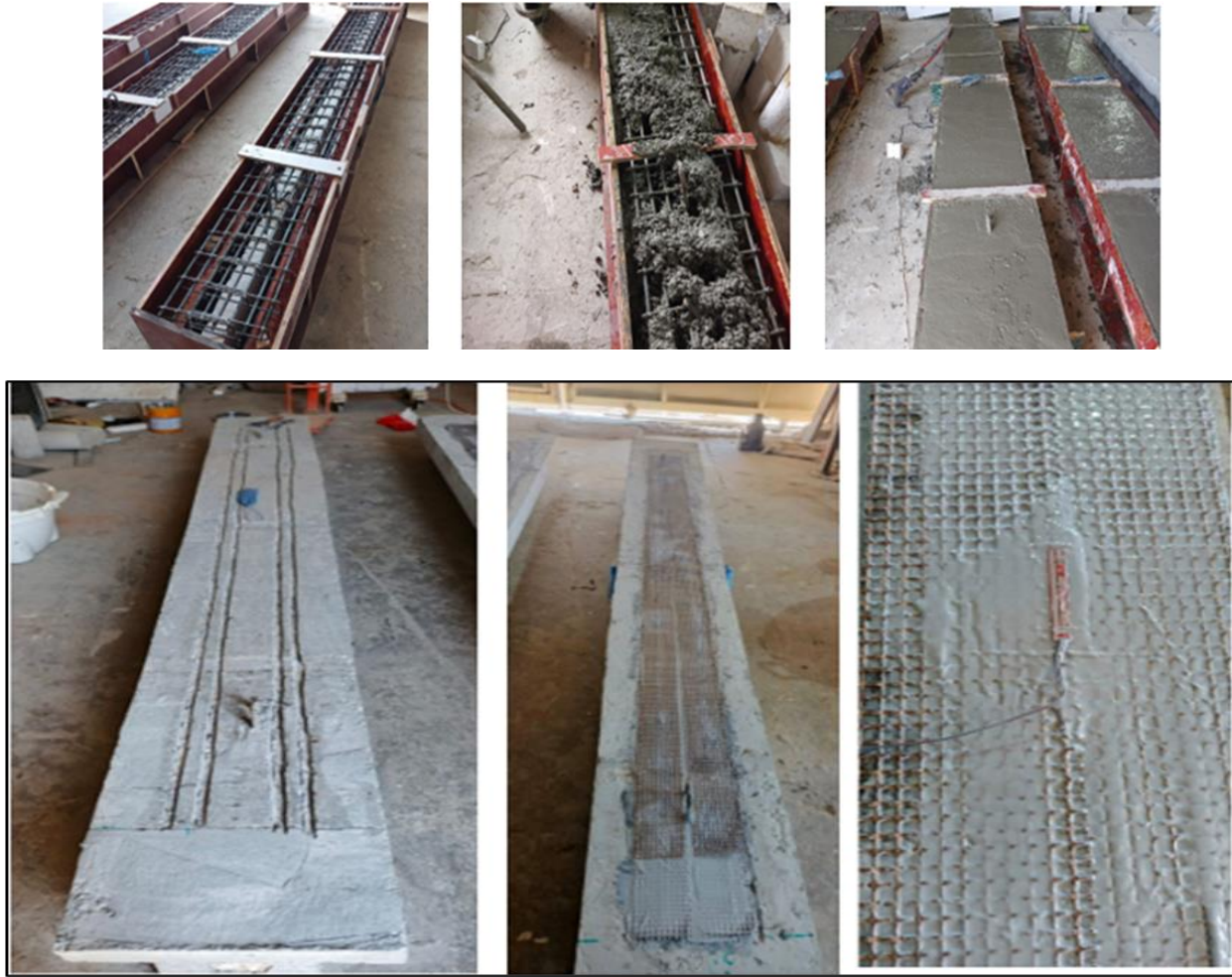
Fig. 9 Preparing of RC T-beams
