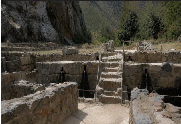
Fig. 7 Outlet sector of the aqueducts running beneath the platforms of the three internal terraces
