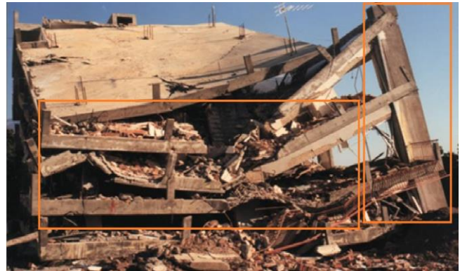
Fig. 7 Progressive collapse of a waffle slab-column system observed after the 1986 Kalamata earthquake (Greece)
