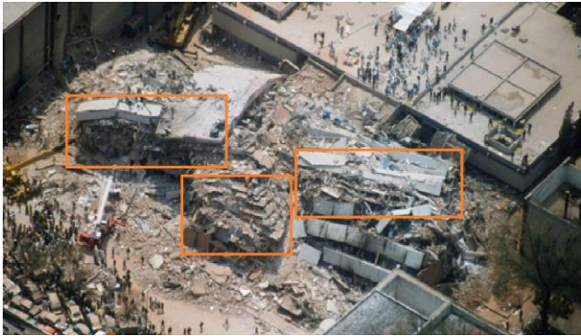
Fig. 1 Progressive collapse of a reinforced concrete waffle slab building (1985 Mexico earthquake.)
