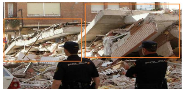
Fig. 4 Pancake-type collapse observed in waffle slab buildings during the 2011 Lorca earthquake (Spain)
