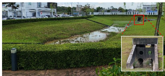
Fig. 1 Example of stormwater detention pond, inlet depicts the pond outlet with a multiple-orifice plate
