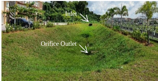
Fig. 3 Selected stormwater detention pond as study area
