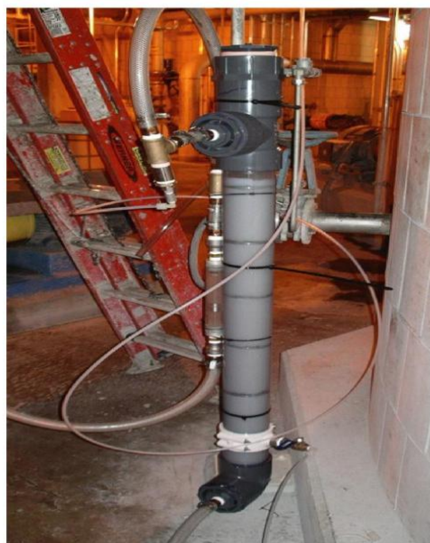
Figure 1: O_3/O_2 aerosol bubble Injection Contact Chamber.
