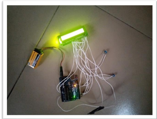
Fig. 2 (b) Arduino, LCD and LM35 temperature sensor powered by a 9v alkaline battery
