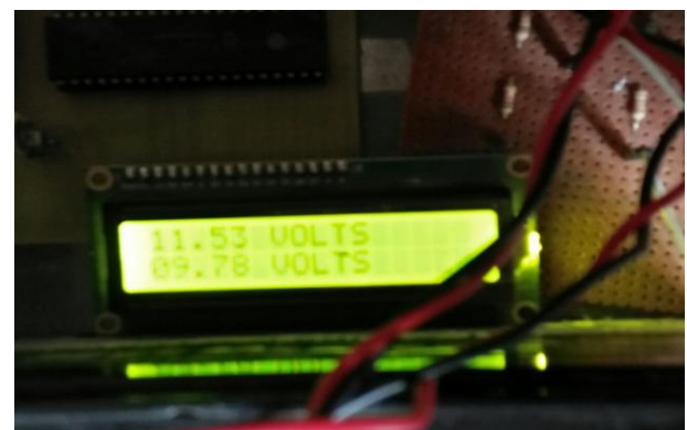
Fig 5 Voltages at Battery
