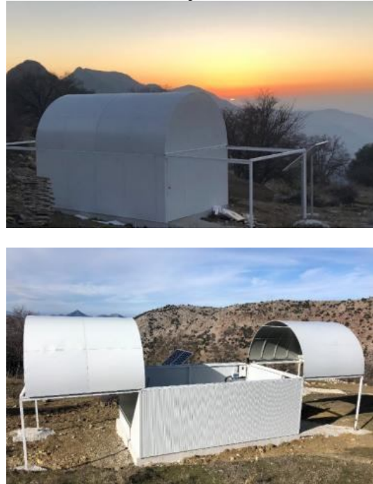
Figure 2. Detail of the vault in Kinsland Observatory closed (above) and opened (below).
