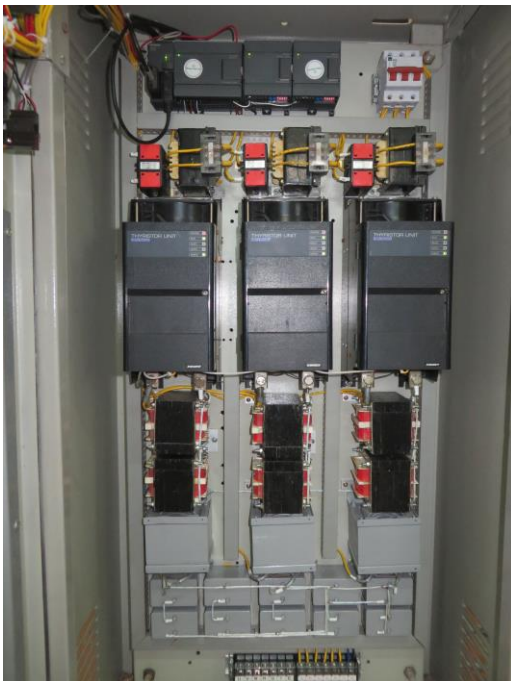
Fig. 8 Real-time PID controller of PLC for SVC
