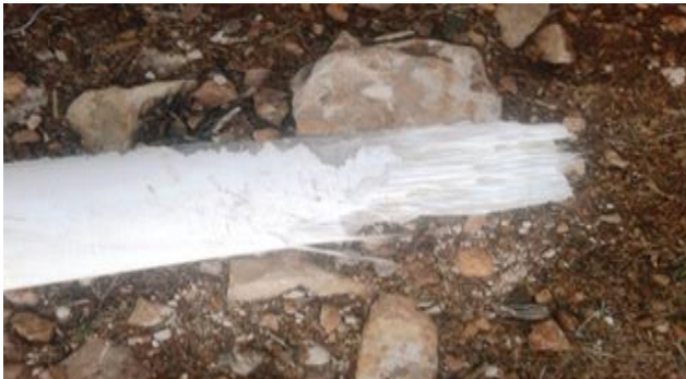
Fig. 9 Mechanical failure at the end of turbine blade
