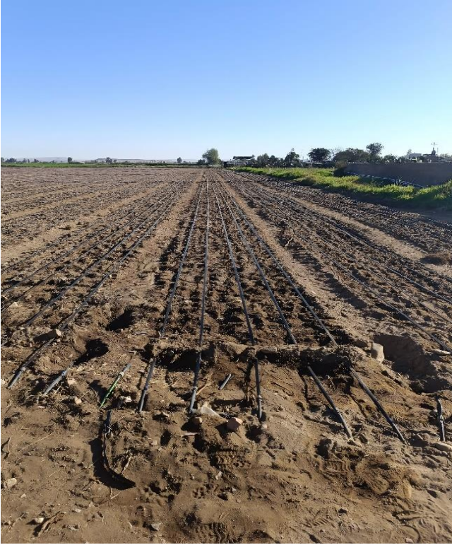
Fig. 3 Piping network for new drip irrigation system
