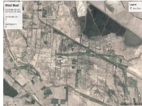
Fig. 1 Shows the aerial view of the wind mast installed at the proposed site
