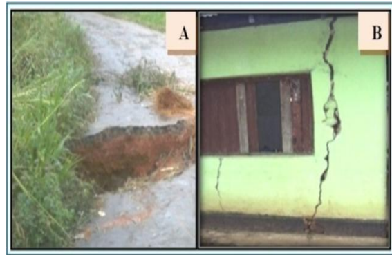
Plate 07: Evidences of soil creep (Kandenuwara–Rattota & SVK division). (Field survey).
