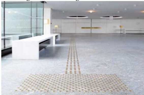
Figure 7 Example of Guiding block Installation. Source: Federal Ministry for the Environment, Nature Conservation, Building and Nuclear Safety (BMUB) (2015).
