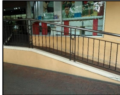
Picture 3.1 Ramp Outdoors
