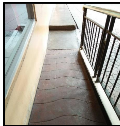
Picture 3.2 Ramp Outdoors
