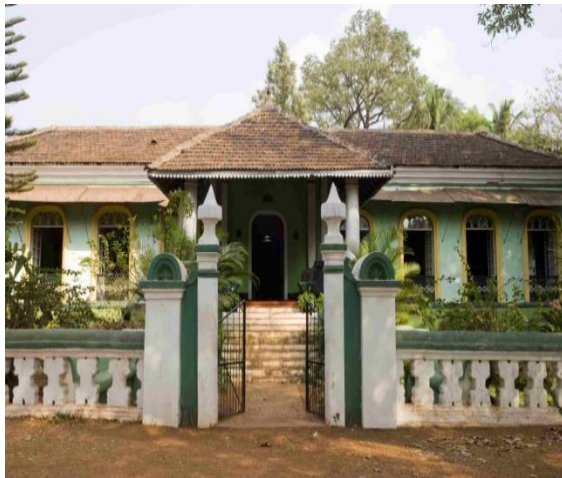
Fig. 6 Restored Portuguese Mansion in Goa
