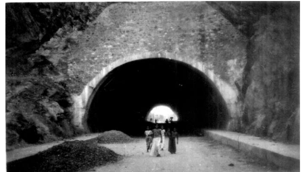
Fig. 13 A tunnel through Indrakeeladri Hill at Vijayawada – 1961
