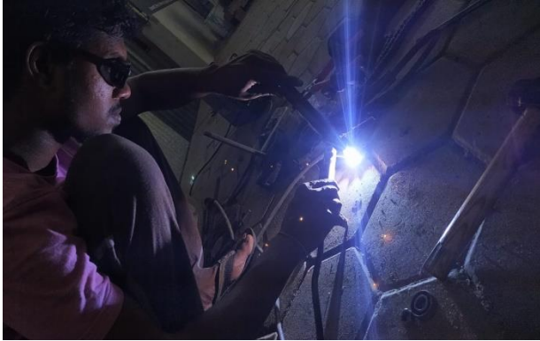
Fig :9 Arc welding
