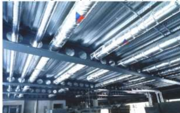
Fig. 1 Passing Pipes Through a Beam With an Opening Web [3].
