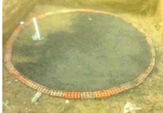
Fig 3 Laying Foundation of the Digester
