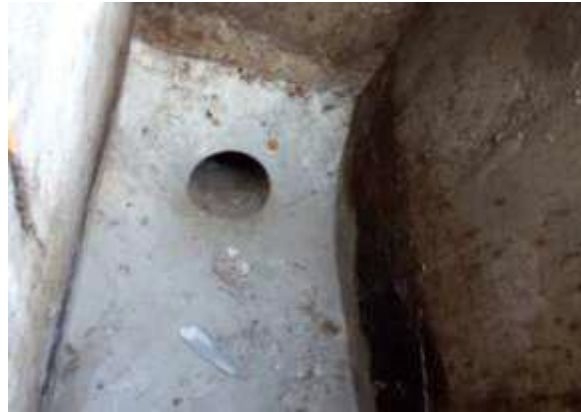
Fig. 5 Inlet Tank With Pipe Passage
