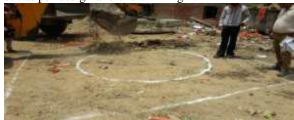
Fig 4 Plant lay-out work
