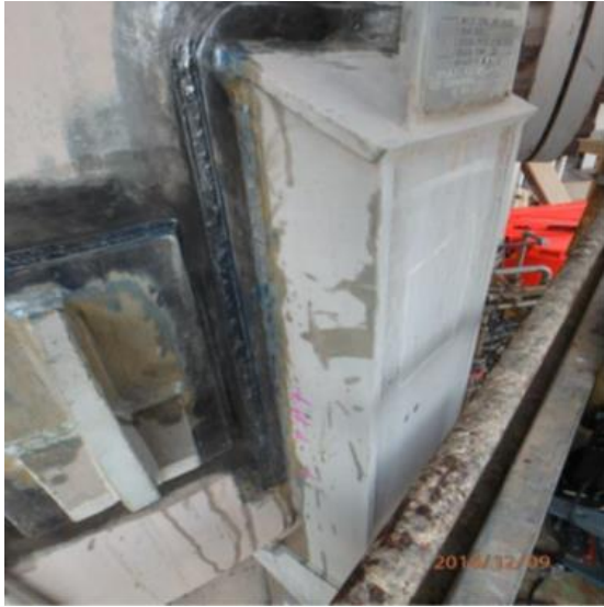
Figure 7 Support leg re-pad weldment
