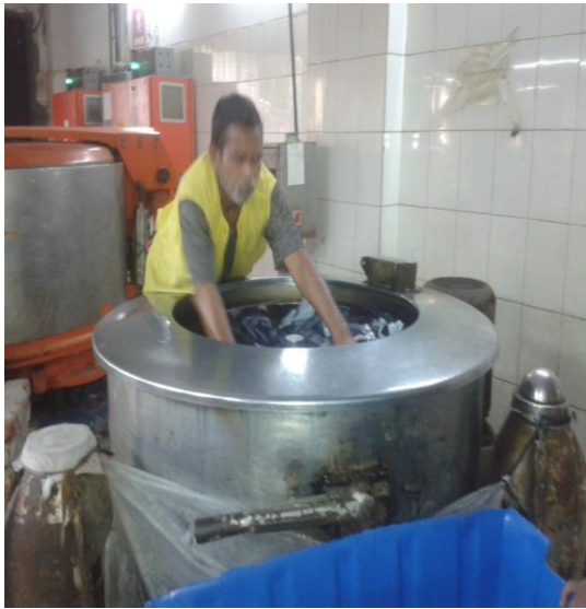
Fig: Hydro extractor Machine
