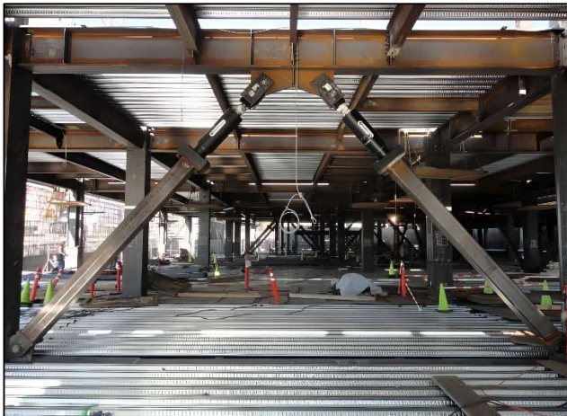
Fig. 5 Viscous fluid damper
