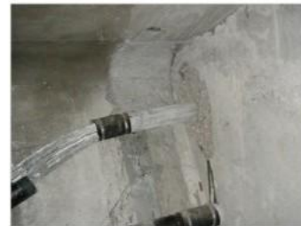
Fig 1.6 Slipping of duct at deviator block
