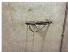
Eruption of PT Tendons caused by Corrosion Failure
