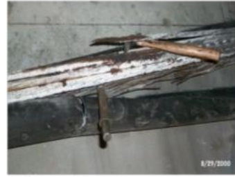
Fig1.5 Cracked duct showing severely corroded strand.
