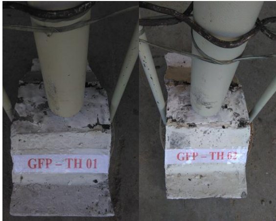
Figure 6. Geopolymer Ferrocement Trough Panels at First crack
