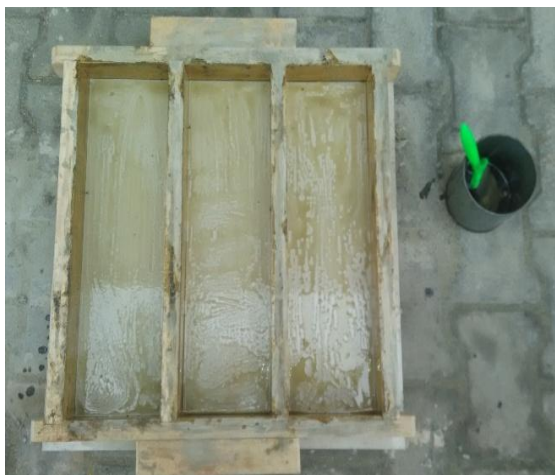
Fig 4: Mould oiled before casting of thickness 20 mm
