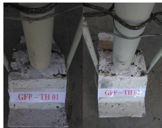
Figure 6. Geopolymer Ferrocement Trough Panels at First crack
