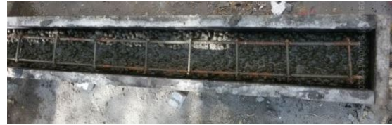
Fig 3: Placing of lightweight aggregate concrete below the Neutral axis
