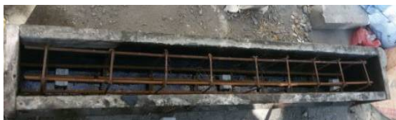
Fig 2: Fixing of reinforcement with cover inside the mould
