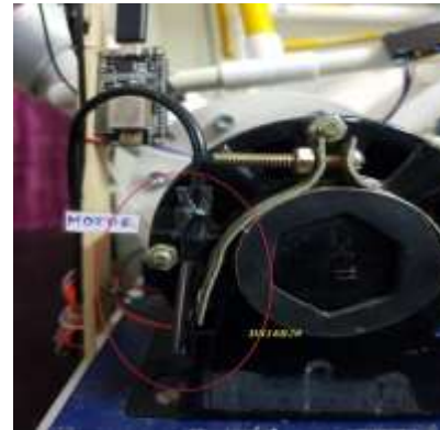
Fig 7:Motor Temperature sensor
