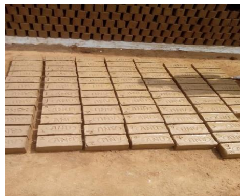
Fig 3 Drying of Bricks
