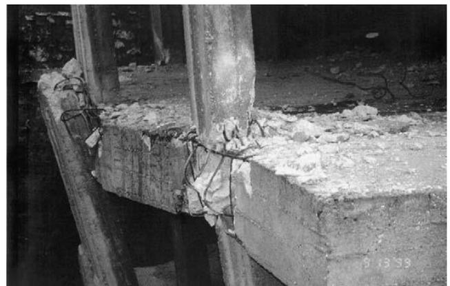
**Figure 2 Typical View of Beam-Column Joint Failure (Reference: [www.researchgate.net](http://www.researchgate.net))**
