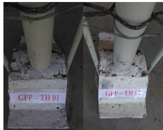
Figure 6. Geopolymer Ferrocement Trough Panels at First crack
