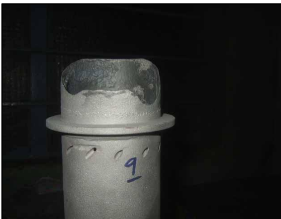
Damaged Crossfire Tube (material erosion/missing at OD)
